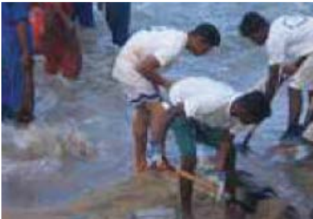
Underwater laying of HDDP pipe line for Lakdhananvi Power Station, Kerawalapityya.
