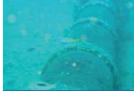
Recovery operation of Old underwater petroleum pipe line With Ceylon Petroleum Cooperation.
