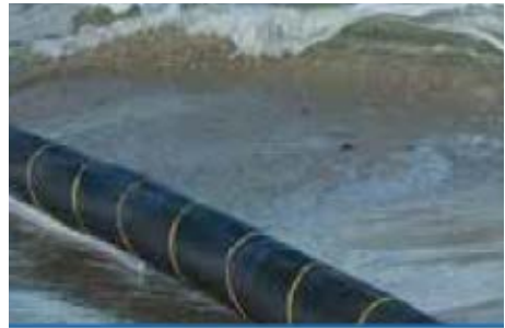
Underwater laying of optical cables (Falcon segment 9.2) – With Alcatel-Lucent
