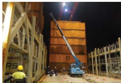
Vessel MSC Daniela Operation - Removal of burnt and damaged cargo to allow dry dock of vessel
